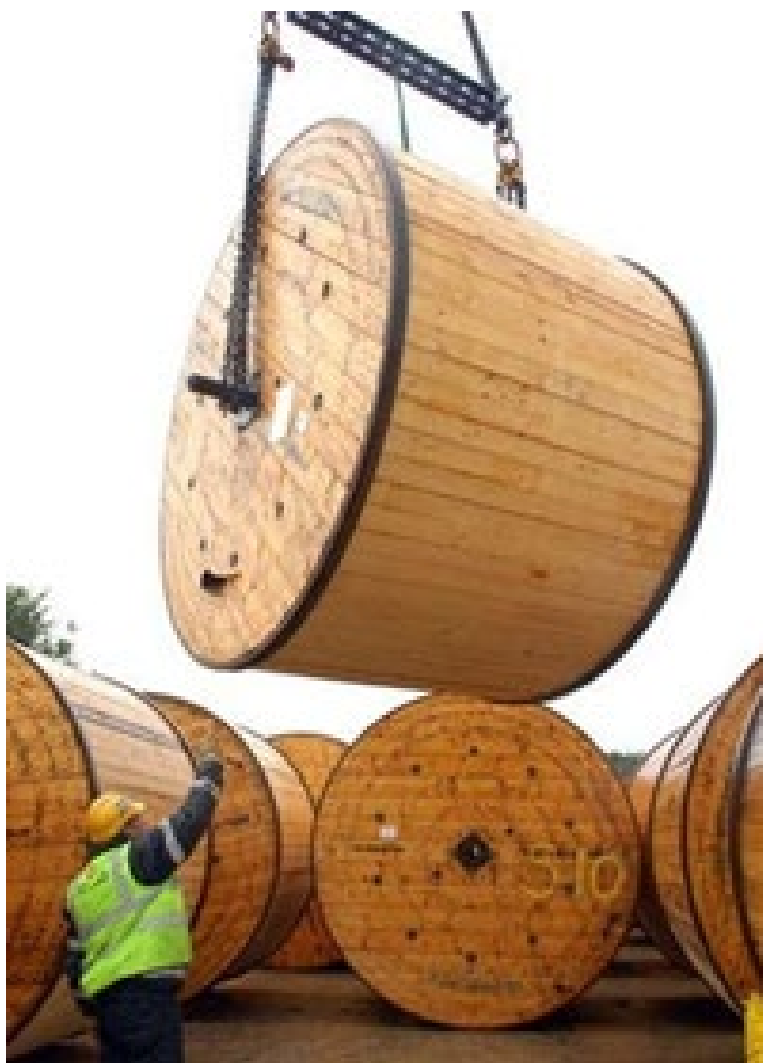
Figure 1.12: Example of a cable drum delivery to cable storage area
